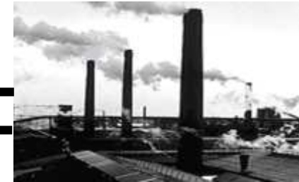
Eskom Coal Based Electricity
